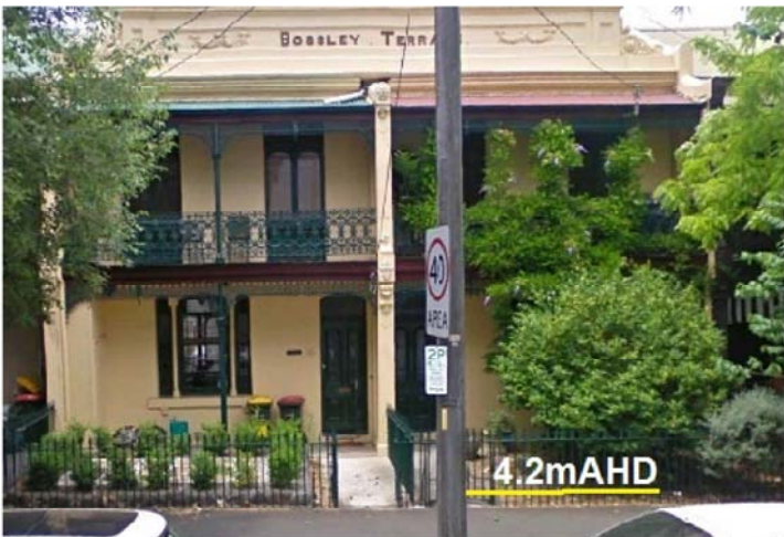
Approximate elevation of regular flooding along front fence outside, 18 Crown St, Woolloomooloo. 4.2m AHD
